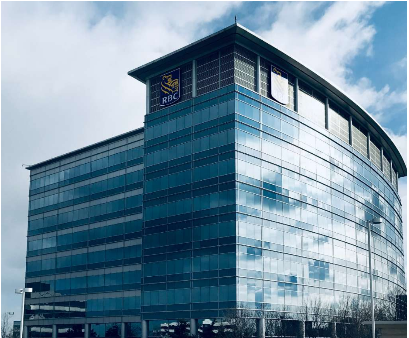
Royal Bank of Canada Head Office, North Side, Canada
